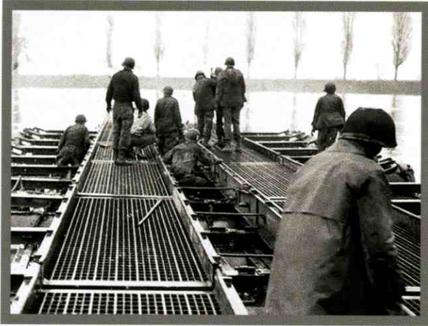
Men of the 36th Engineers work during combat to construct a float bridge during the Second World War. (Above photo courtesy of the author. Title page photo entitled "Bridge from the Berlin Side" was provided to the author by Allison Chmielewski who is the daughter of 297th Engineer Combat Battalion veteran Al Hutchings)
